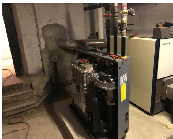
Pose chaudière, Ecole Koechlin
